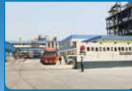
位於江蘇泰興的溶劑廠房 The solvents plant in Taixing, Jiangsu
