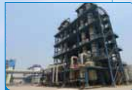
位於廣東江門的溶劑廠房 The solvents plant in Jiangmen, Guangdong
