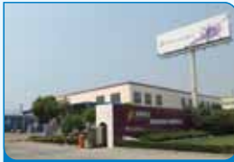
位於上海青浦的塗料廠房 The coatings plant in Qingpu, Shanghai
