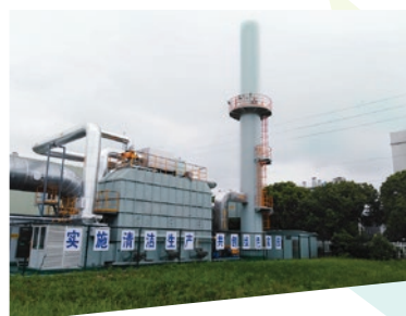
桐鄉油墨廠房的VOC處理設施 Tongxiang inks plant's VOC treatment facility
